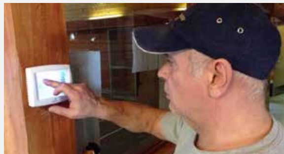
The AEA's Tom Gross installing a programmable thermostat in a home in Jean Marie River.
