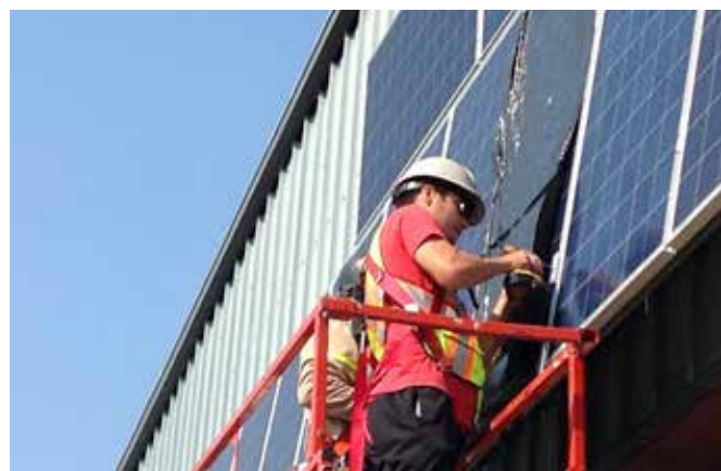
A contractor installs solar panels on the recreation centre in Fort Simpson.
