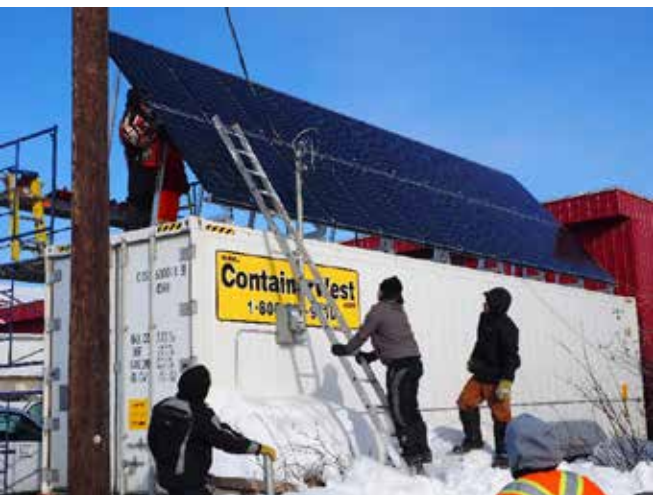
Installing solar panels to power the Inuvialuit community freezer in Inuvik.
