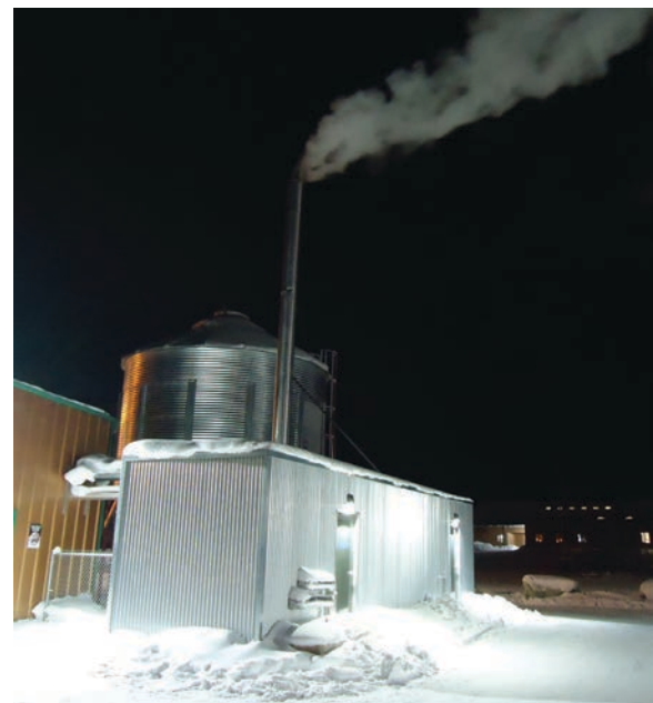
The container for the pellet boiler that powers Whati's district heating system, with the pellet silo in the background.
