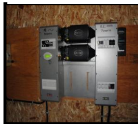
Two 3.6kW inverters in shed
