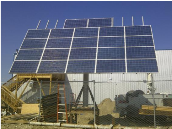
Pole mounted system in Behchoko. Photo credit: Ventek Entreprises
