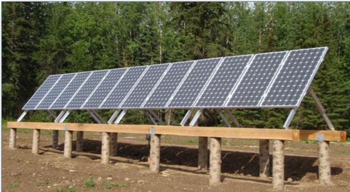
2.1 kWp low-profile PV mount.
