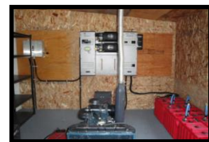
Eight batteries in shed
