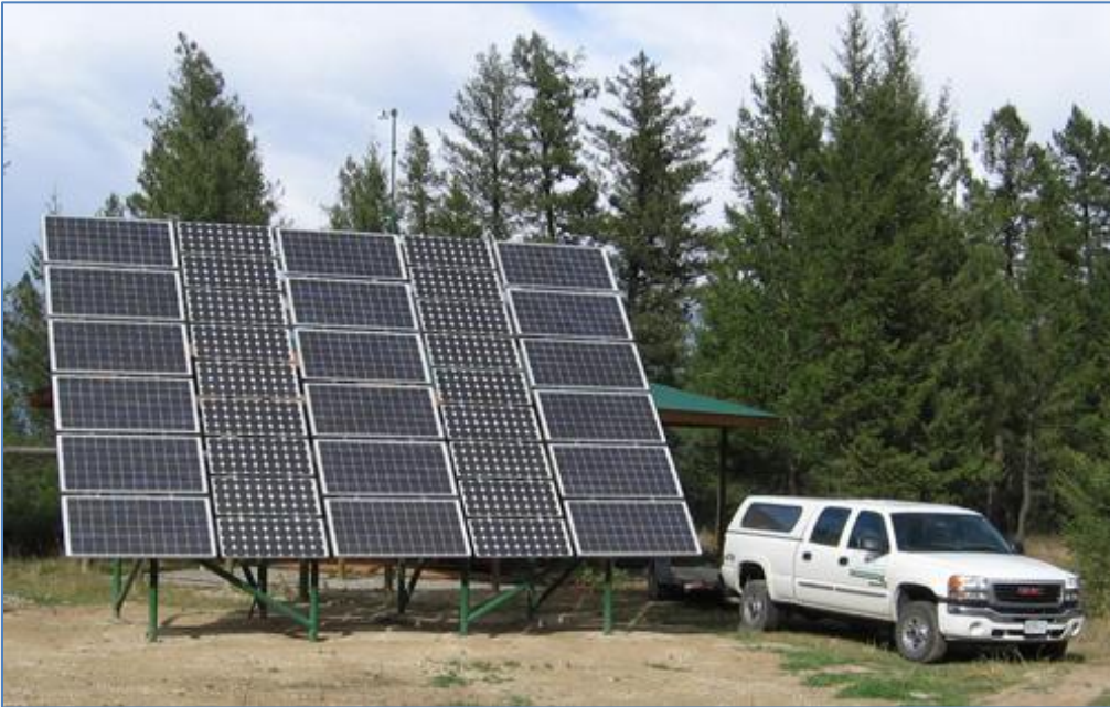
2.1 kWp low-profile PV mount.
