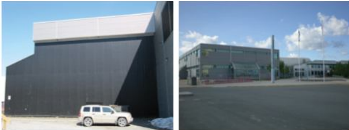
Figure 2. SolarWall at Weledeh Catholic School, Yellowknife
