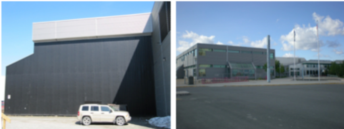
Figure 2. SolarWall at Weledeh Catholic School, Yellowknife
