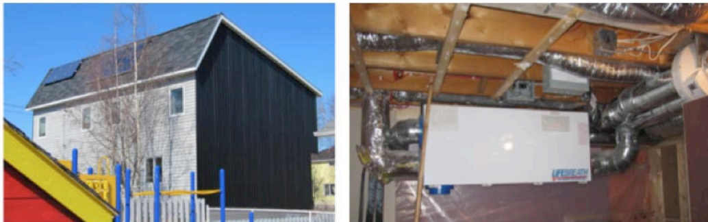
Figure 4. SolarWall façade on a private house, Yellowknife
