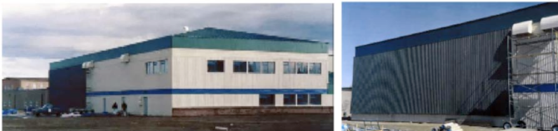
Figure 5. SolarWall at Fort Smith Recreation Center, Fort Smith 60°N, Picture from Conservall Engineering (2010a, b)
