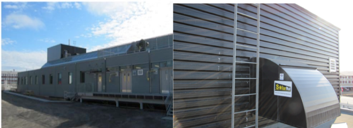
Figure 7. Aurora Research Institute, Inuvik; Left: Back of building with SolarWall on the Penthouse; Right: Close-up of the SolarWall;
