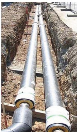
Photos: Finnish Forest Research Institute. Left- Lengths of pre-insulated pipe. Right- Trenched Pipe.
