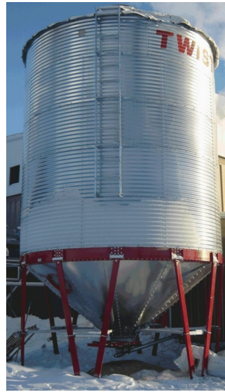
Left Photo: AEA. Welded steel plate silo. This 40t silo is 8.2m tall, diameter of 3.7m Right Photo: AEA. Bolted corrugated steel sheet silo. This 55t silo is 8.2 m tall, diameter of 4.3 m
