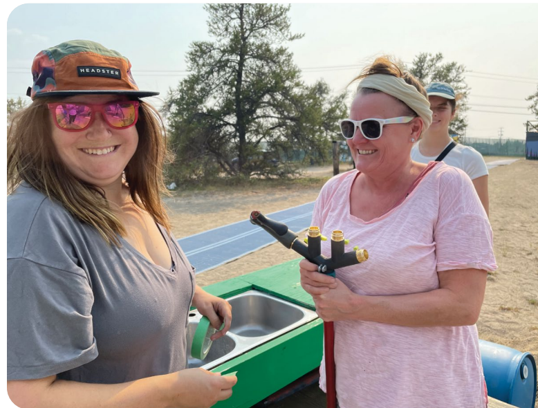
Every year we use renewable energy systems to provide hot water for Ecology North's dishwashing station at Folk on the Rocks in Yellowknife. And sometimes when gear doesn't work like it should, we need to come up with creative solutions on the fly.
