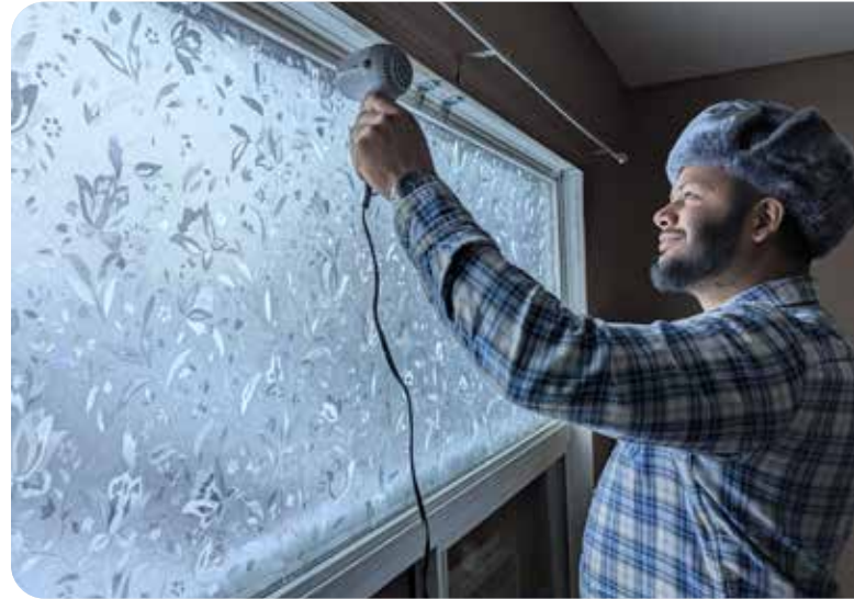
A homeowner applies window plastic as part of our Home Winterization Walk-Through pilot in Yellowknife.
