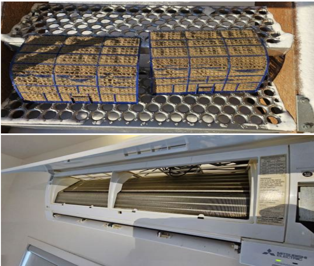
Dirty filter from Unit A (top) and missing filter from Unit C (bottom).
